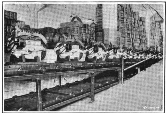
Fig. 21—The Willlys-Overland Co. has a motor storage department on the opposite side of a roadway from the building containing the motor assembling department. Motors are carried over into this storage department on an apron-type conveyor which runs through a tunnel under the road. This conveyor was built and installed by the Link-Belt Co., of Chicago, Ill.
